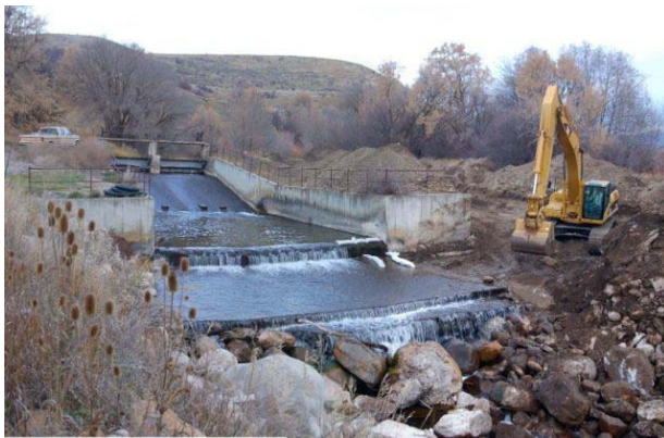
Bypass channel construction at Cub River, Idaho diversion site in 2006.
