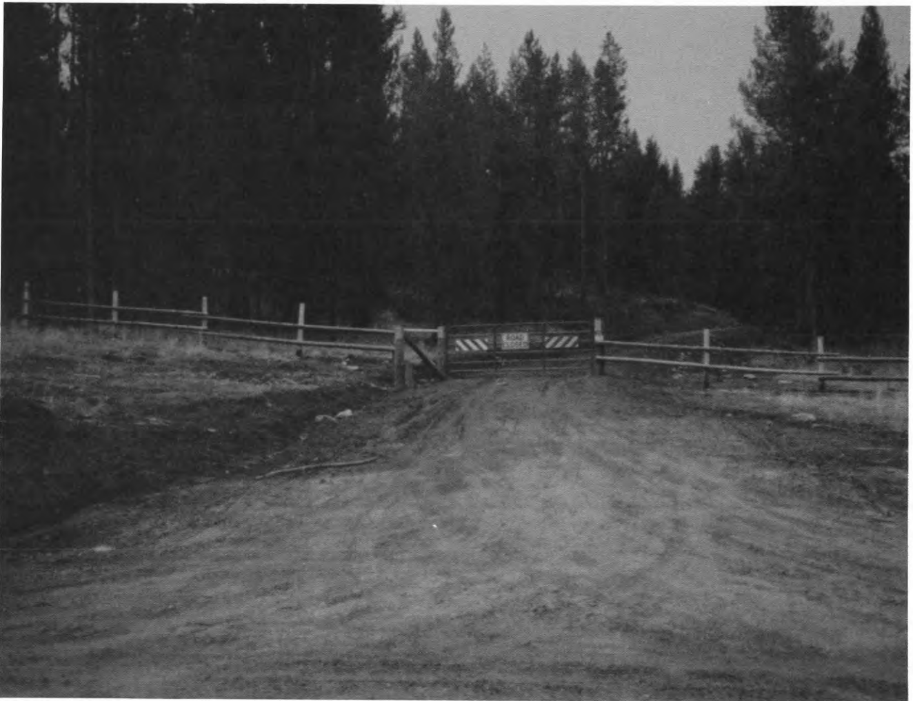
Gating new roads following timber harvest provides security for wildlife while retaining the road for future management needs, Targhee National Forest.
