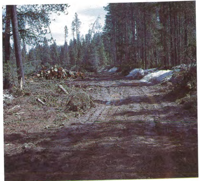
Low standard "work roads" such as this one on the Targhee National Forest will be obliterated and reseeded following the timber sale.
