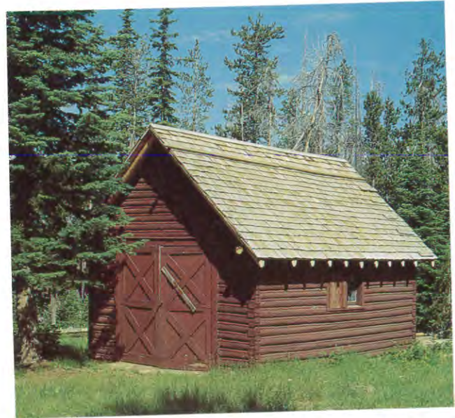
Management of cultural resources can take several forms. The new roof on the garage at Bishop Mountain Lookout, Targhee National Forest, retains the building's unique characteristics.
